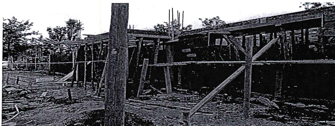
Ongoing Construction of 400 student capacity dormitory at Aquinas High School.
