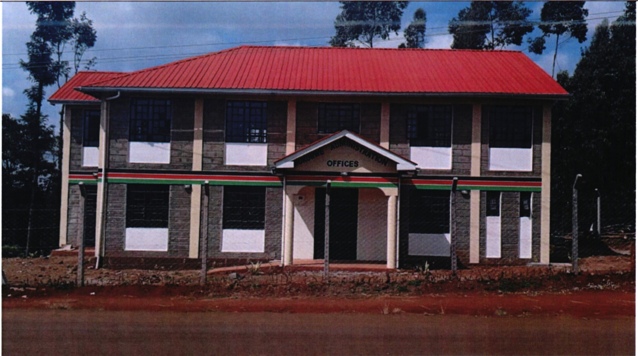
Construction of 7 number Mukurwe Chiefs office (The project expected to enable administrative and other government extension services to approximate population of 29,243 residents of Mugumoini ward)
