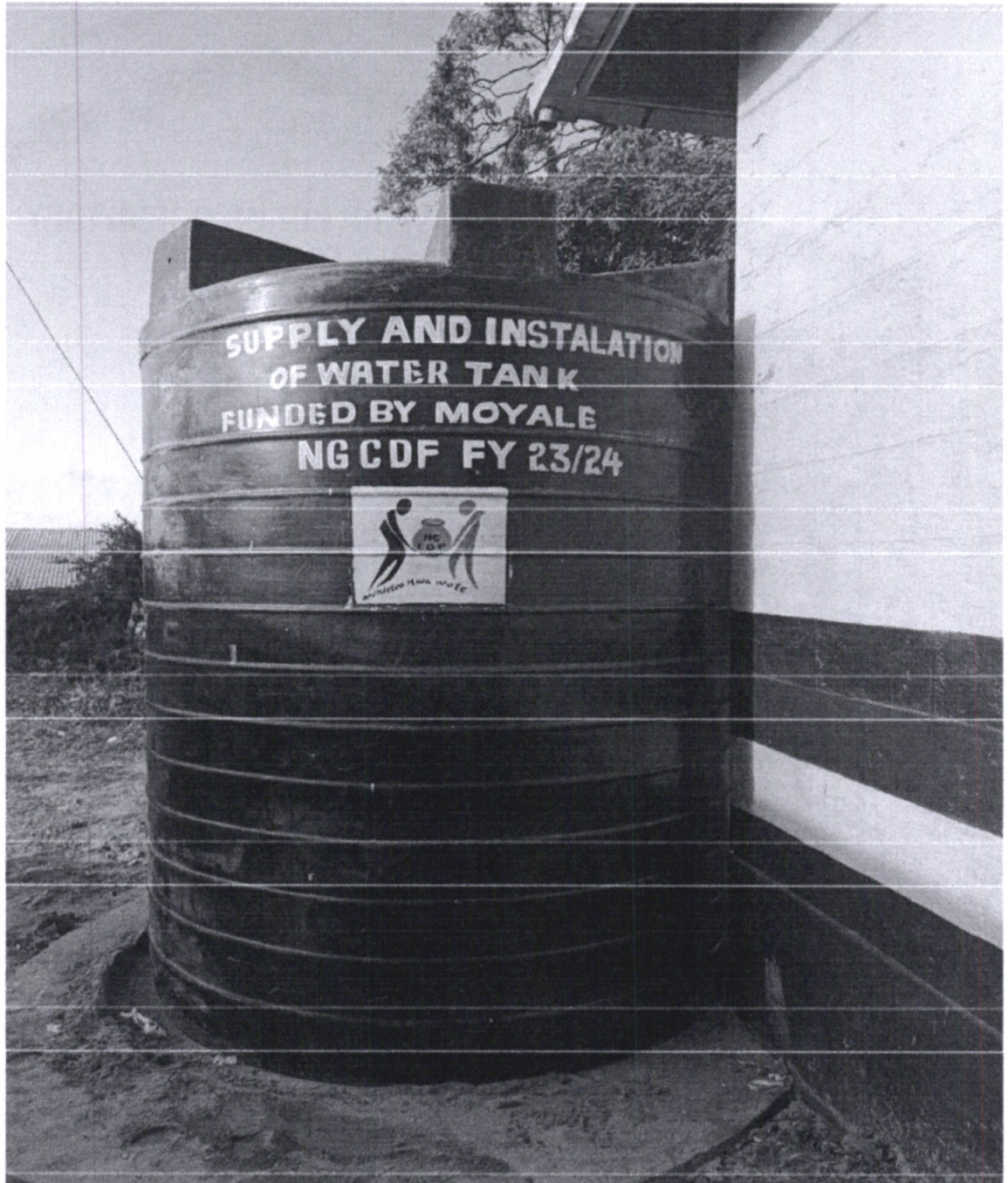
Installation of water Tank and gutters at Moyale police division H/Qs
