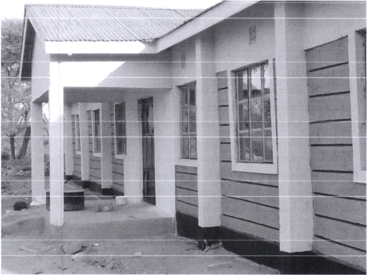
Construction of Dormitory at URAN Secondary school
