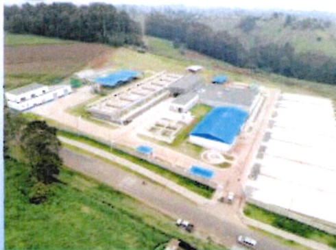
Aerial Photo of completed Kigoro Water Treatment Plant
