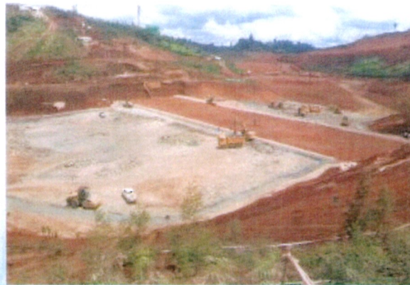
Ongoing Dam Filling works – Karimenu II Dam Project
