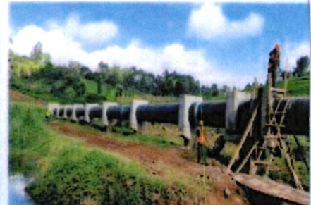
Aerial Crossing for NCT Pipelines project
