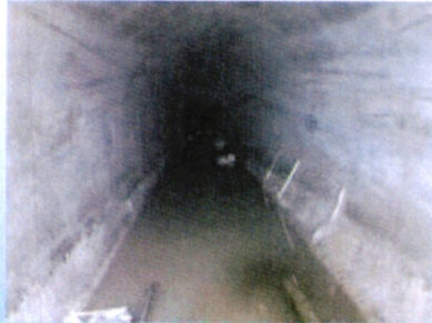
Lined Tunnel - Northern Collector Tunnel (NCT) Project
