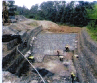
Githika Outfall Gabion Laying - (NCT)
