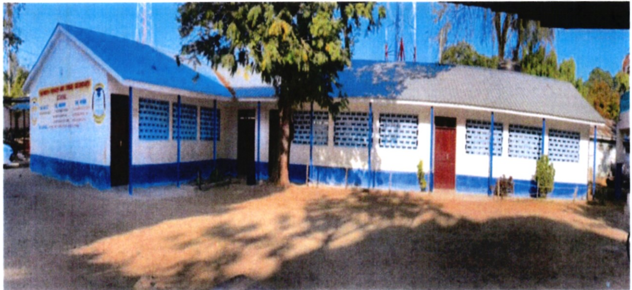
Construction of four classrooms at Tom Mboya Primary School in Mombasa County.
