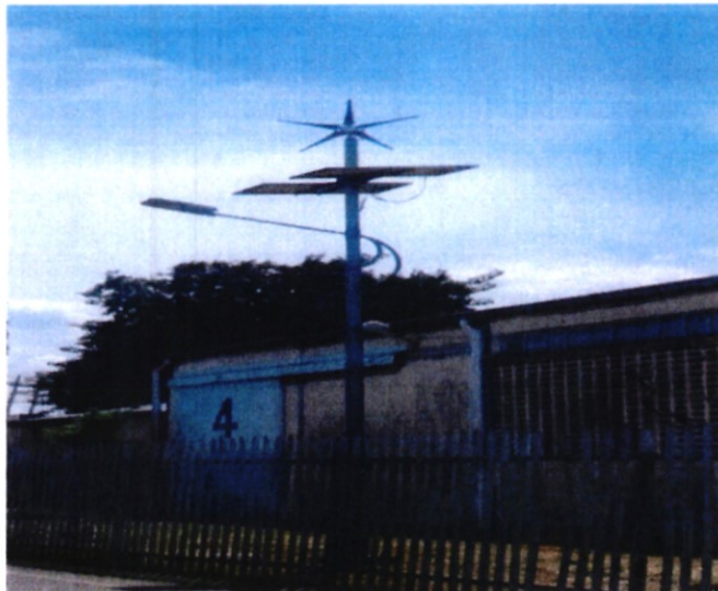
Wind and solar energy lighting
