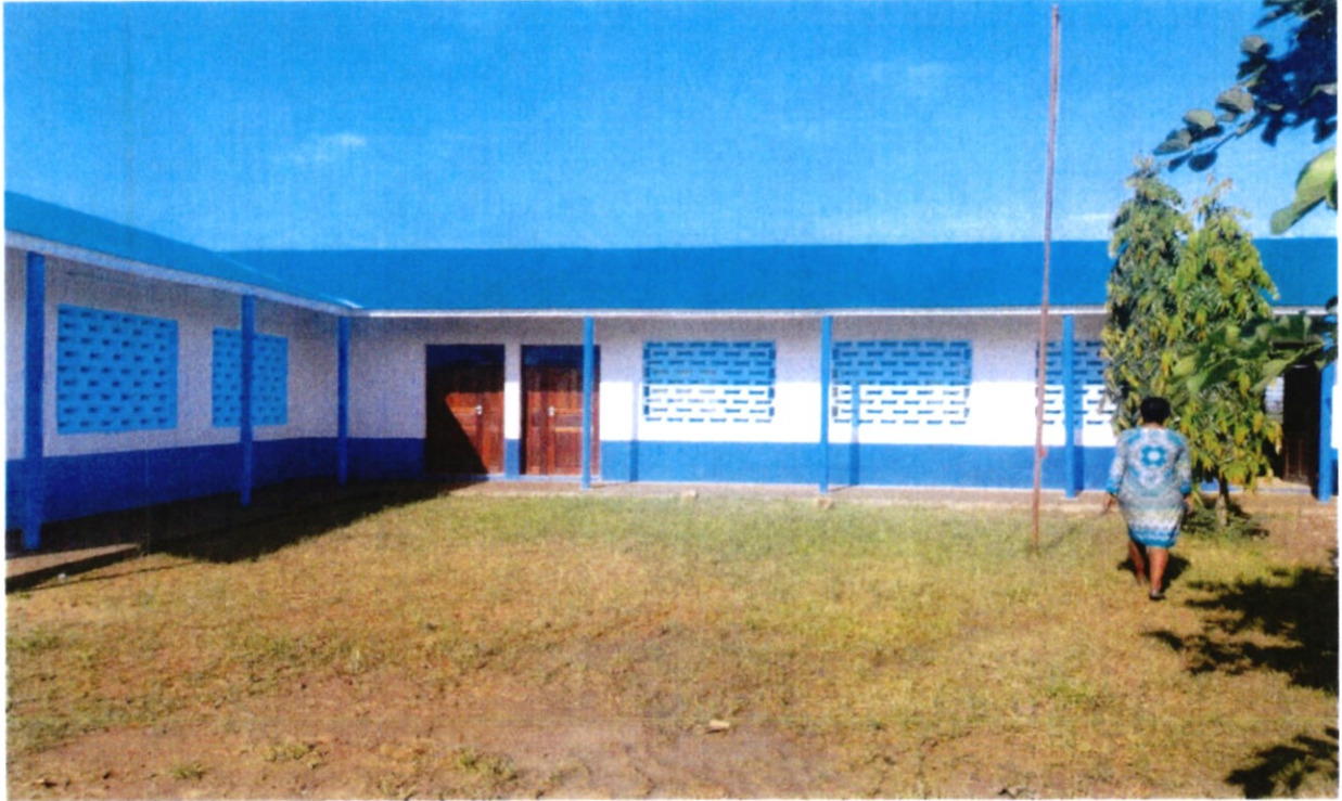
Baraka Voroni Primary in Mombasa County construction of four classrooms.
