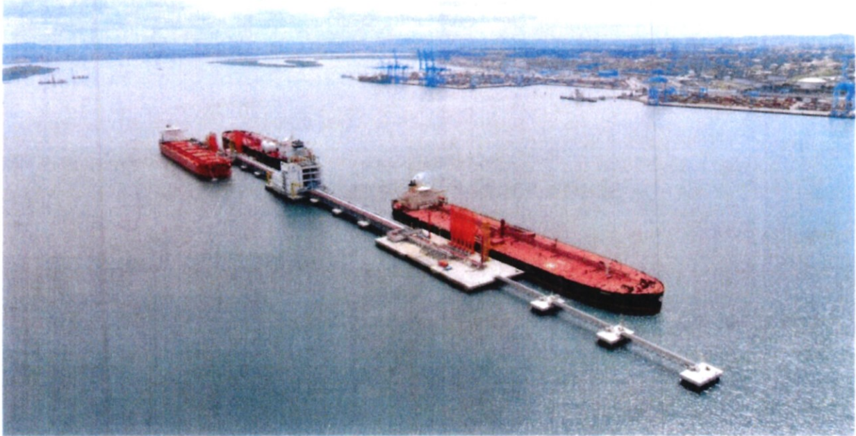
New Kipevu Oil Terminal (KOT II)
