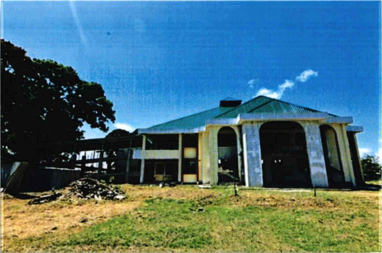
Miritini Rehabilitation Center under construction
