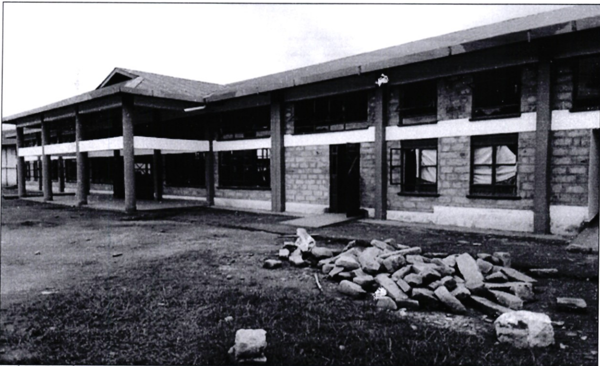
Kobujoi Police station construction of the station
