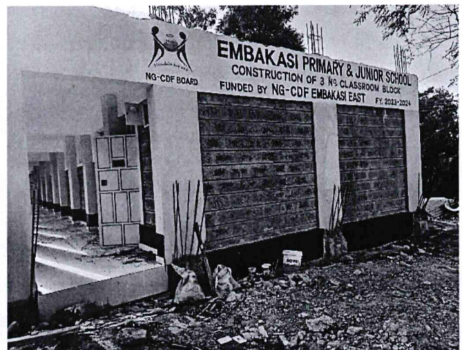
3No Classrooms at Embakasi Primary School
