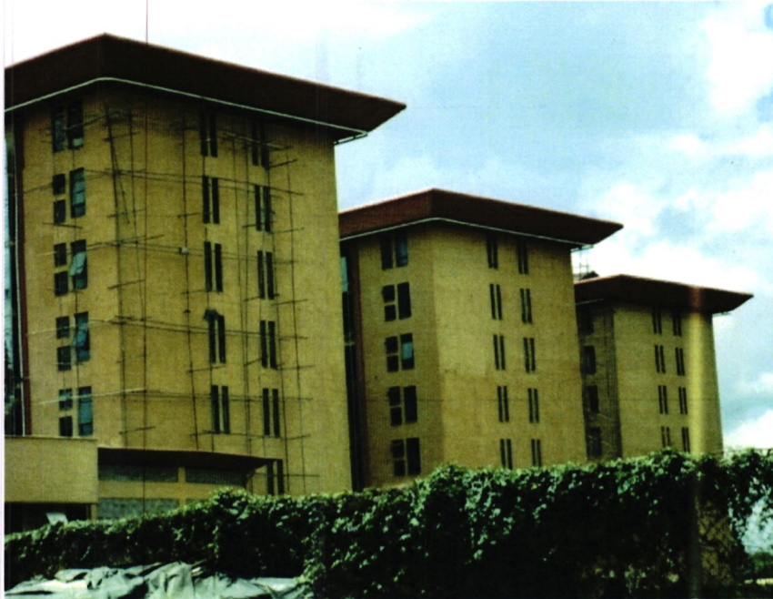
The New Mitihani House (Ongoing Project)
