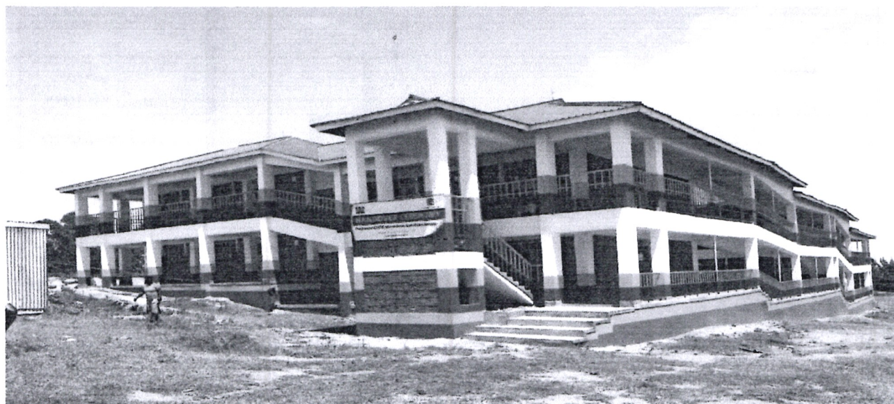
KMTC Navakholo – Construction of Storey building of 12 lecture halls in Bunyala Central Ward, complete and handed over but final payment will be done in 2021/2022 FY
