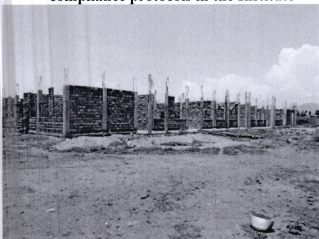
Construction of proposed Mbita technical and vocational training college at Waondo in Mbita constituency being mentored by Mawego TTI
