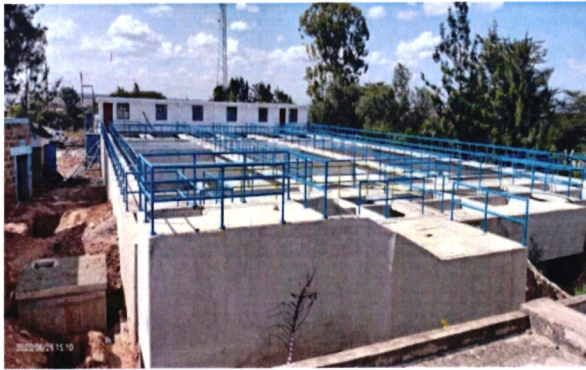
Mavoko Drinking Water Project Water Treatment Plant
