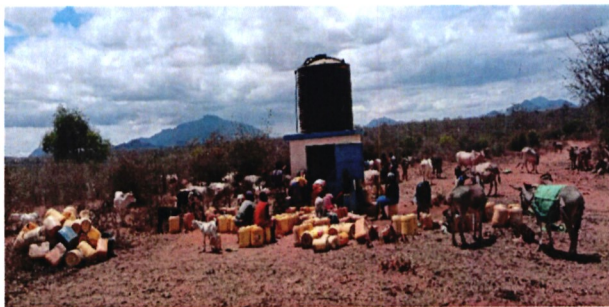
Wananchi taking water from Kaluasi Borehole Water Project constructed under the Drilling & Equipping 40No. Boreholes funded by GoK
