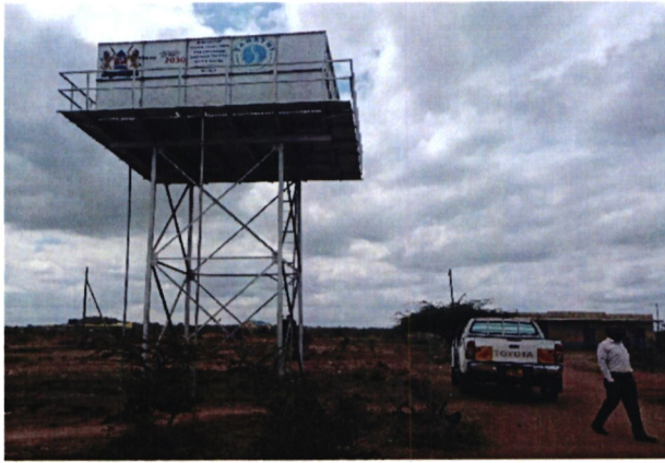
Masinga-Ikaatine-Ekalakala Water Project - Elevated tank at Kanyonyo market centre
