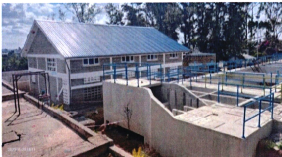
Mavoko Drinking Water Project- WTP_Chemical Building and Mixing Chamber
