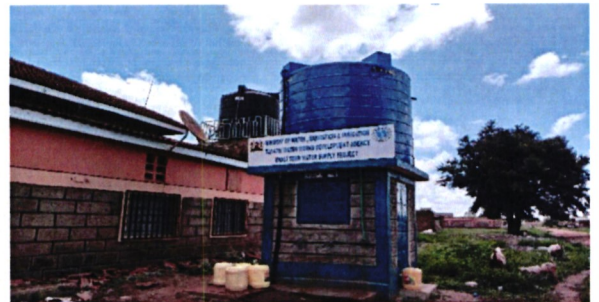
One of Water Kiosks for Emali Water Supply Project
