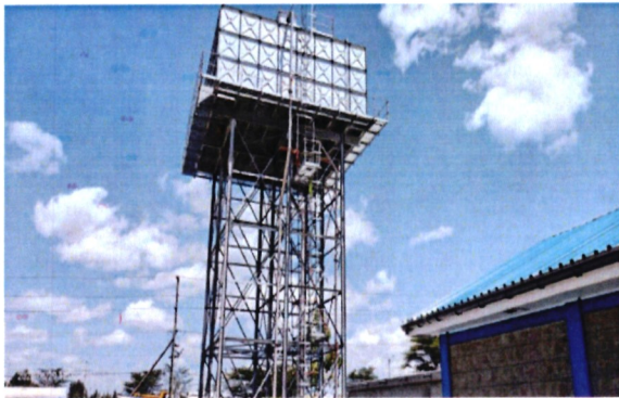
Mavoko Drinking Water Project- Syokimau_300m3 Elevated tank
