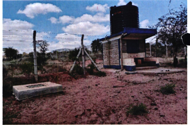
Nuu Special School Water Kiosk Constructed under drought mitigation programme
