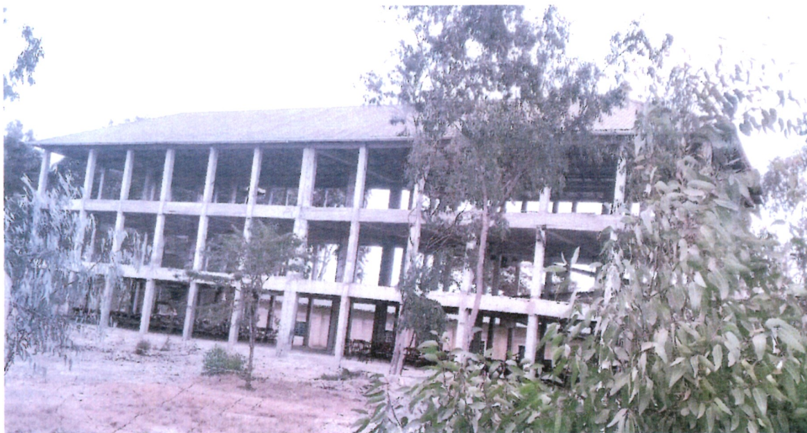
Figure 1 Completed Phase 1 of Electrical and Electronics Workshop Funded by MOE
