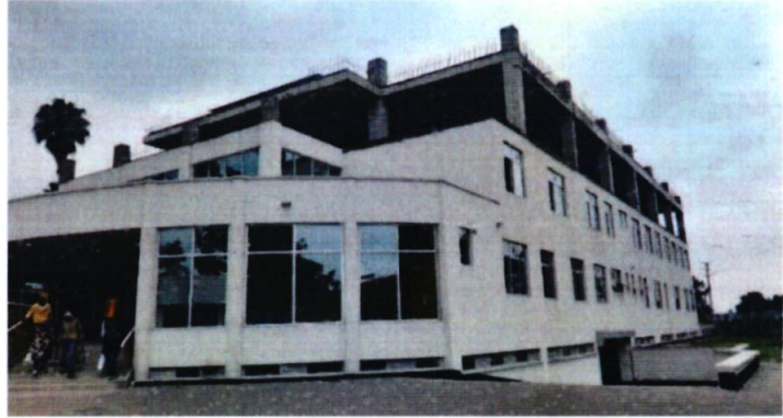
Phase 1 CTC complete and operational
