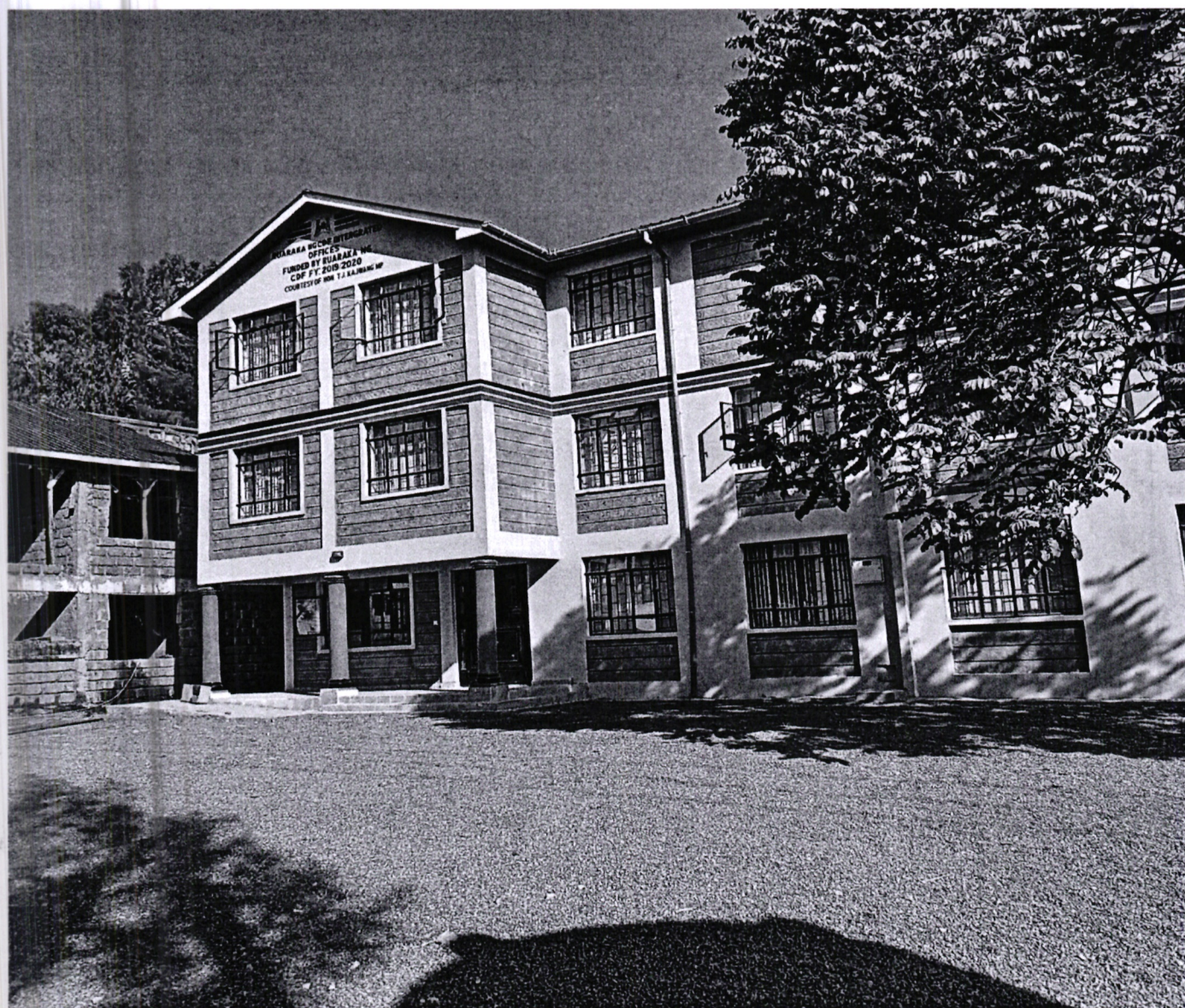
Figure 3: Construction of Intergrated Ruaraka NGCDF Office
