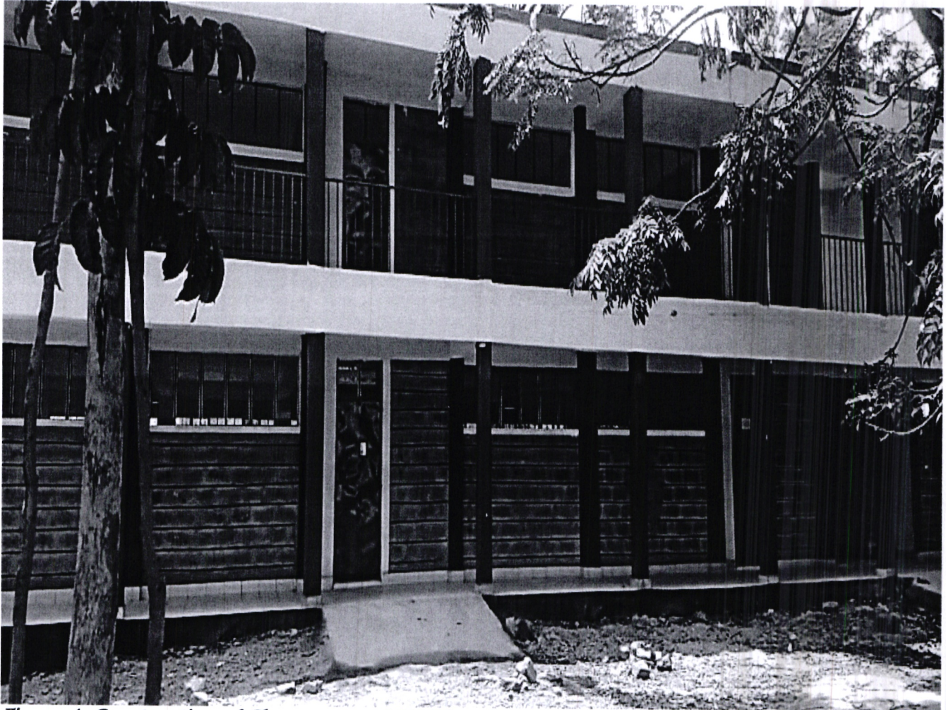
Figure 4: Construction of Classrooms at MM Chandaria Primary School
