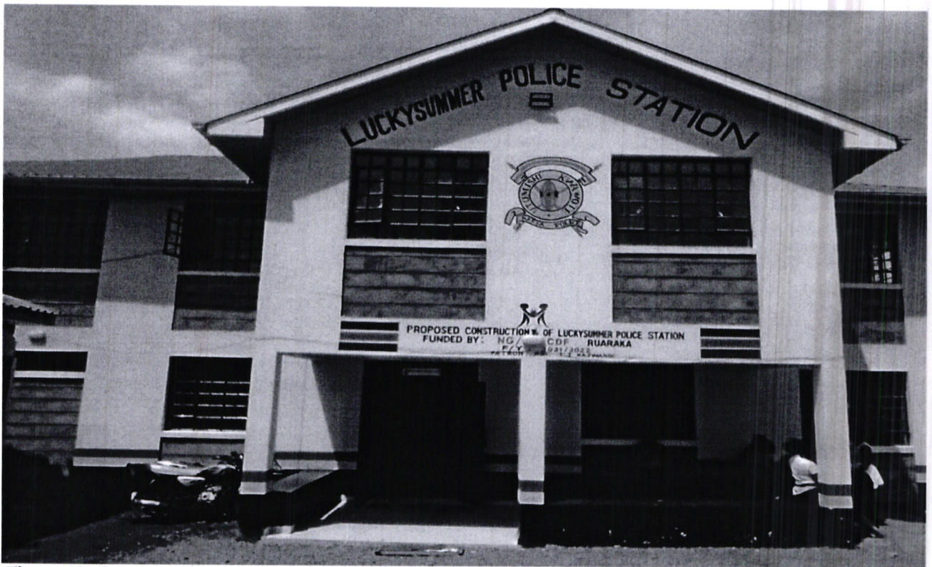
Figure 2: Construction of Lucky Summer Police Station
