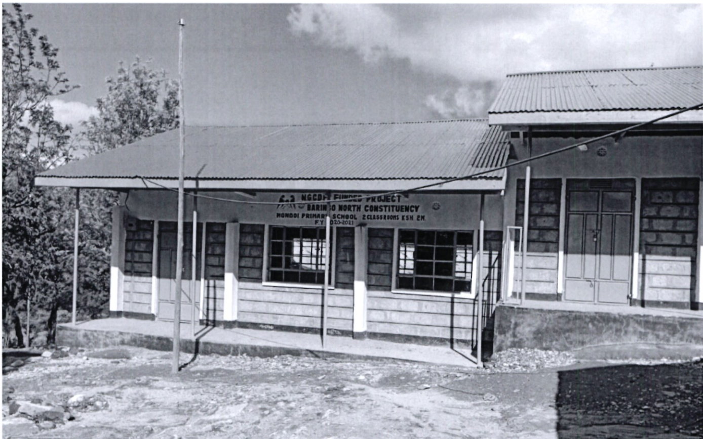
Mondoi Primary School – Construction of Two Classrooms
