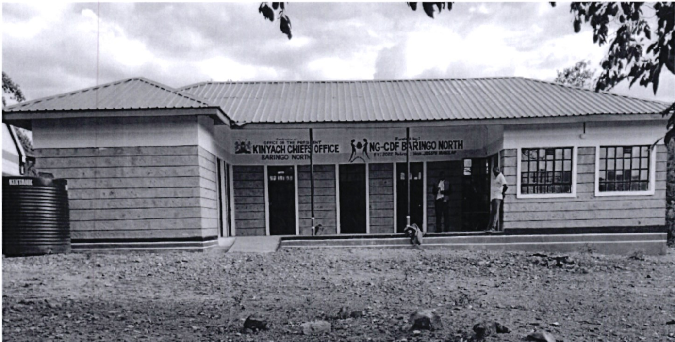
Kinyach Chiefs Office – Construction of Chiefs Offices
