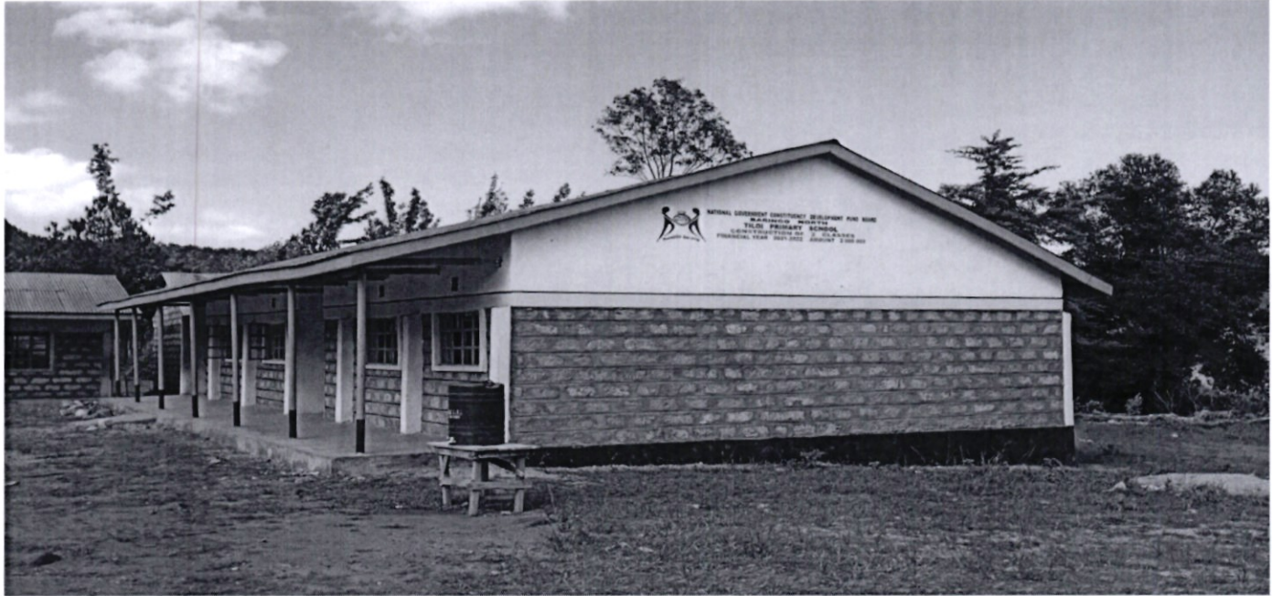
Tiloi Primary School – Construction of Two Classrooms
