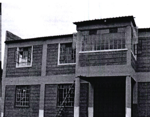
Figure 2: Ongoing Kariga Mixed Secondary School
