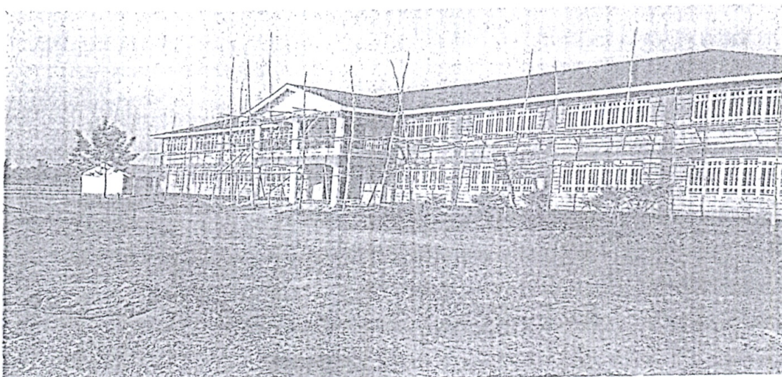
Fig 3: Mundika Secondary School completion of a storey Administration Block consisting of 5 offices, staff room, computer room with capacity of 40 computers and a library; internal finishes, tiling and painting.
