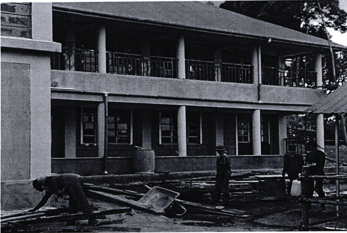
Figure 1: Entanda Primary school – Construction of 8 Classroom on a storey building.
