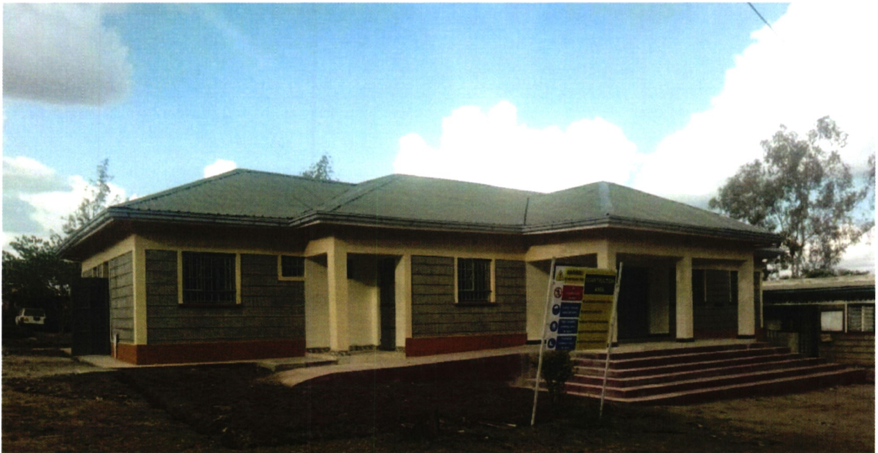
Newly constructed Samburu Office
