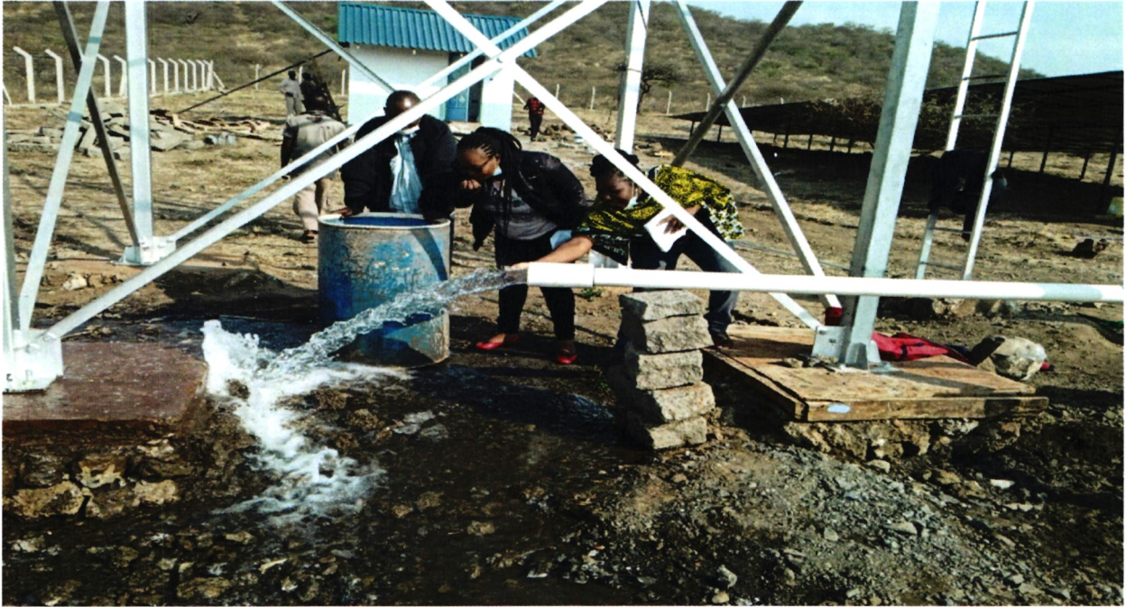
Water borehole at Challa
