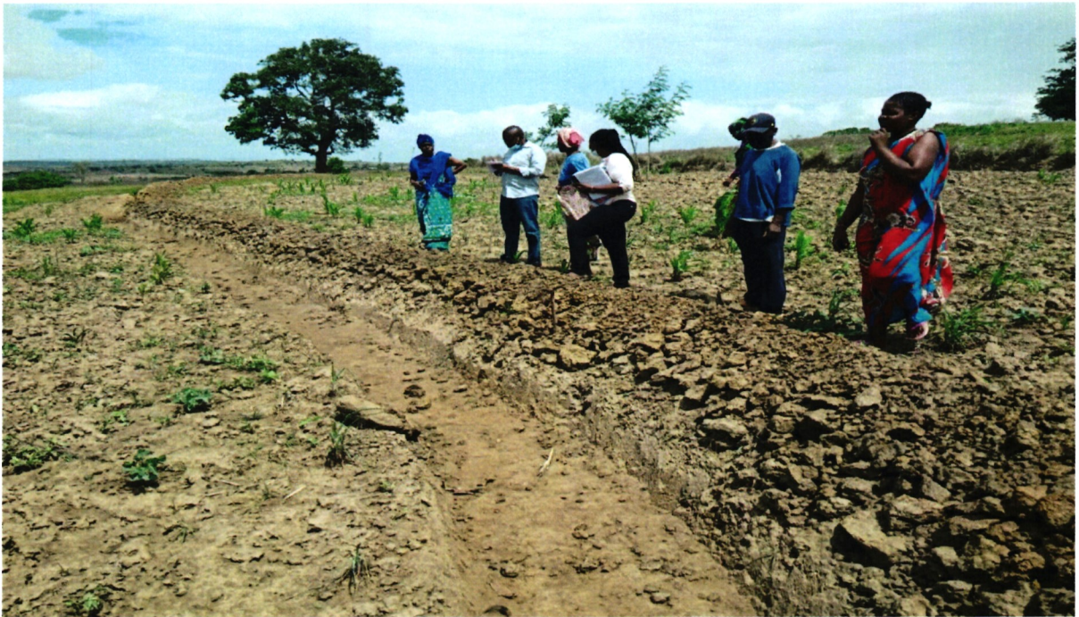
Ongoing terracing work at Mwache
