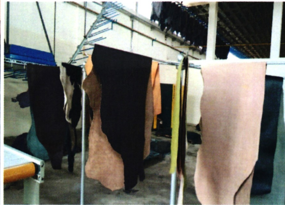
Installed overhead dryer
