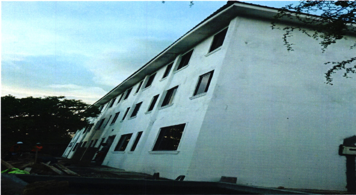
Newly constructed conference facility at Kilifi
