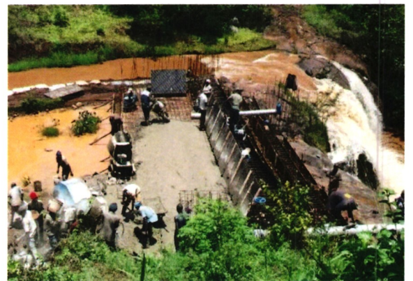
Gaitega Gatari project-River diversion works during intake structure construction
