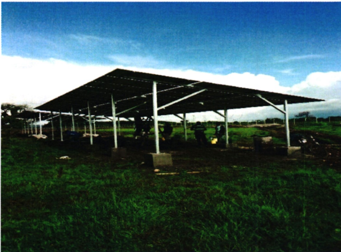
Solar array installation and mounting at Lichota Integrated Technology Transfer Centre
