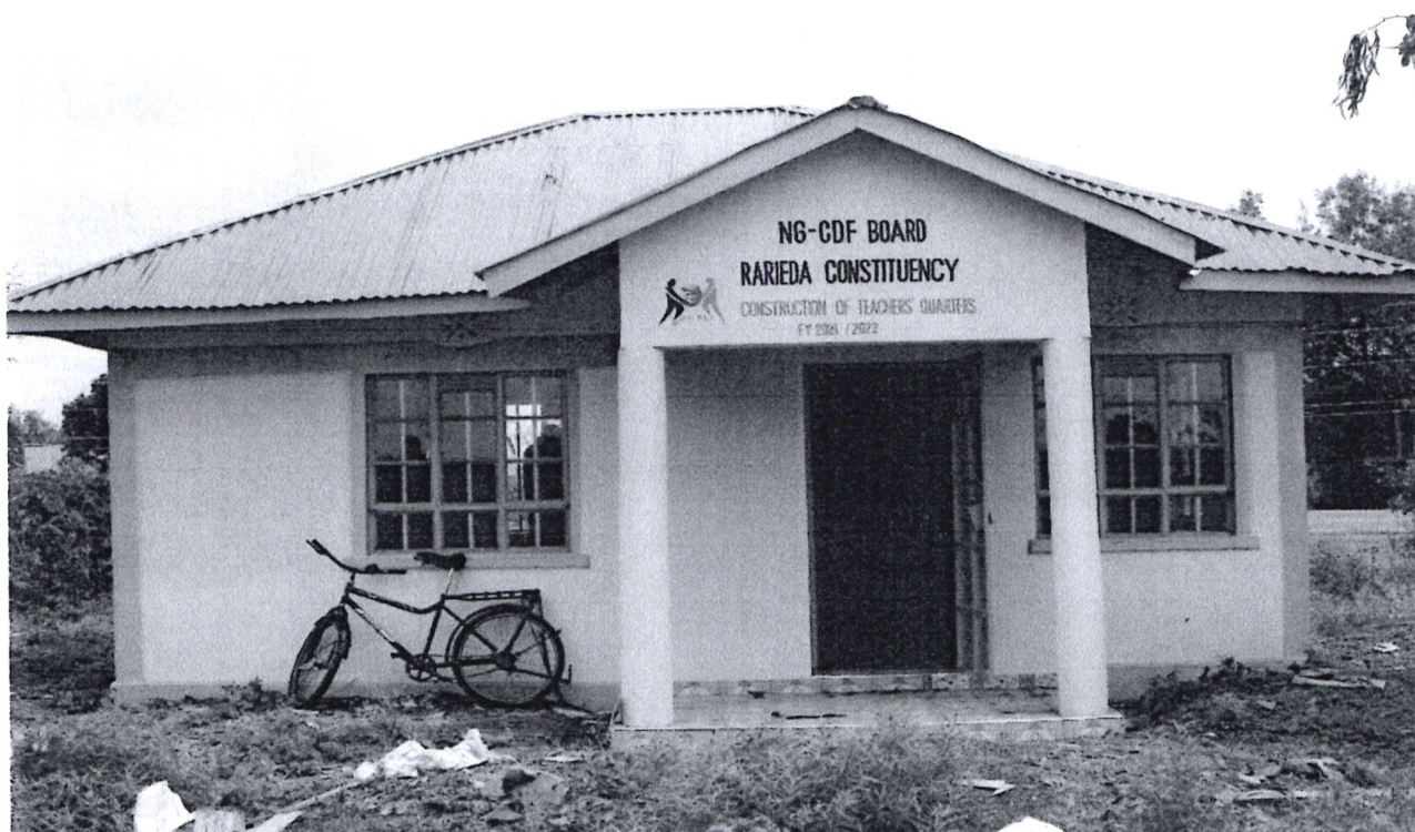
Figure 3: Chianda Primary School, Completion of a 3 roomed staffs quarters.
