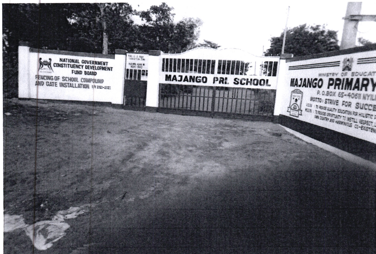
Figure 6: Fencing and Installation of a Gate at Majango Primary School.
