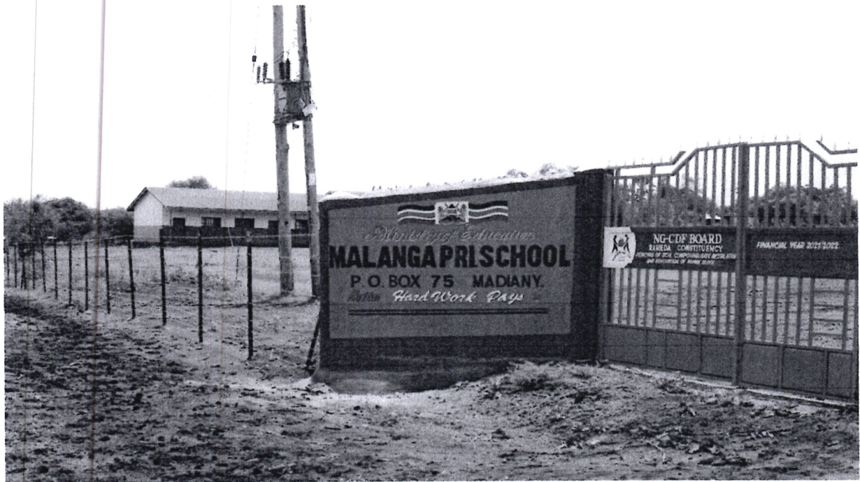
Figure 5: Fencing and Installation of a gate at Malanga Primary School.
