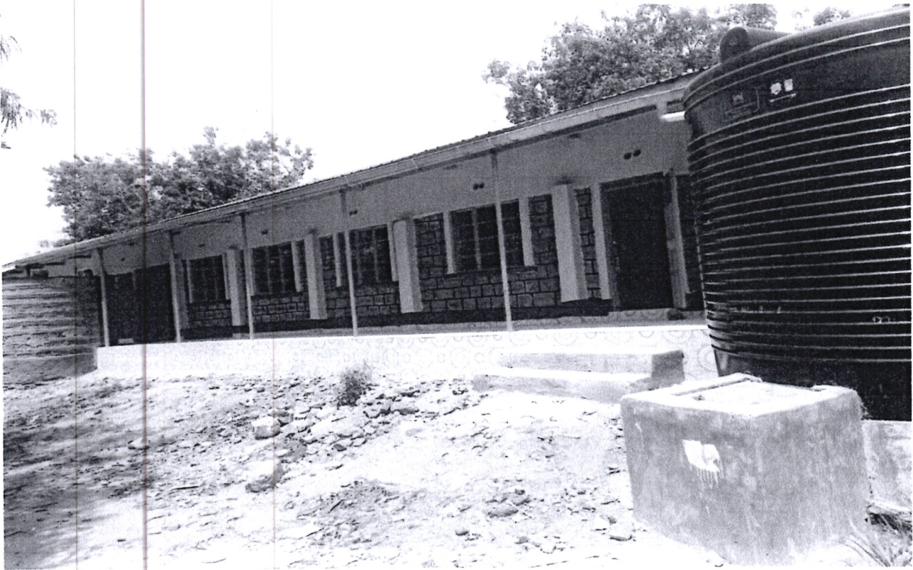
Figure 1: Mirau Primary School, Completion of two classrooms, Front View.
