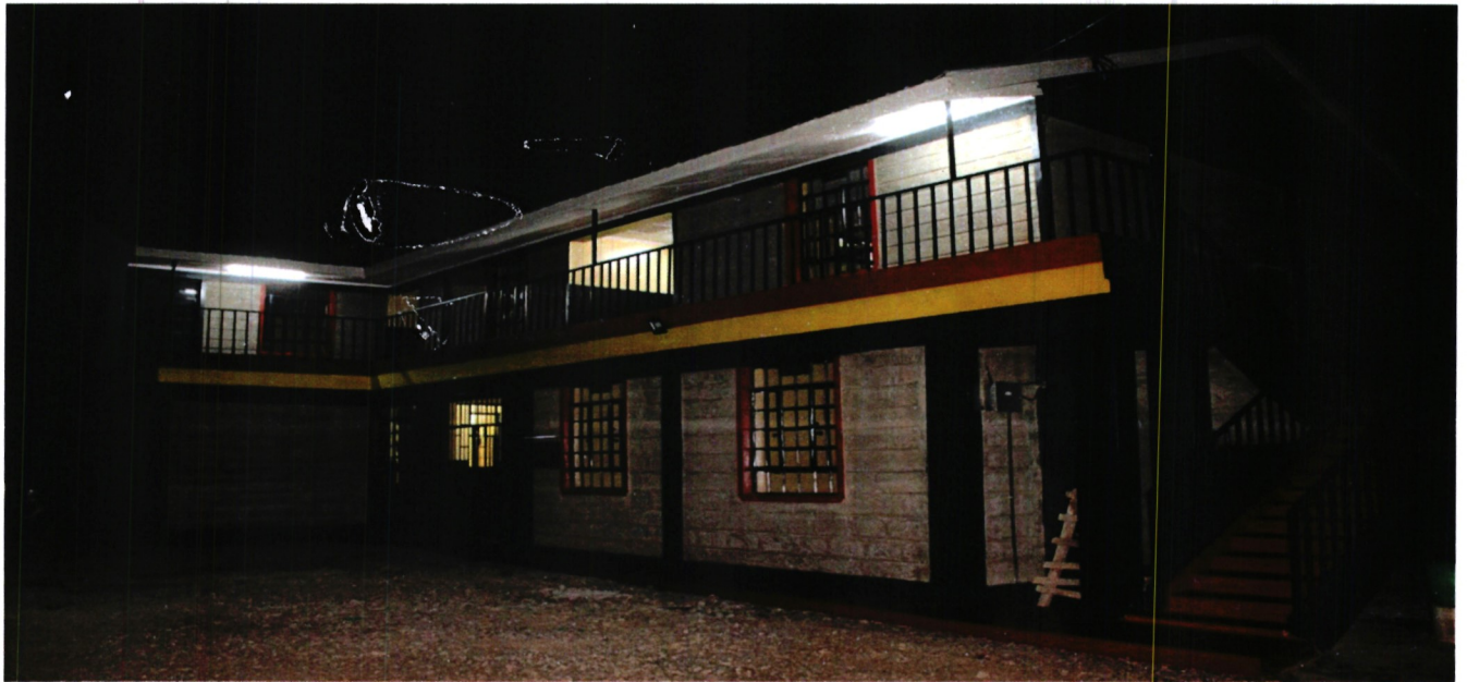
Construction of 8no office, 3no cells and a waiting area post for Kirwara Police Station (The project expected to enable administrative services to the approximate population of 18,000 residents of Gatanga ward)
