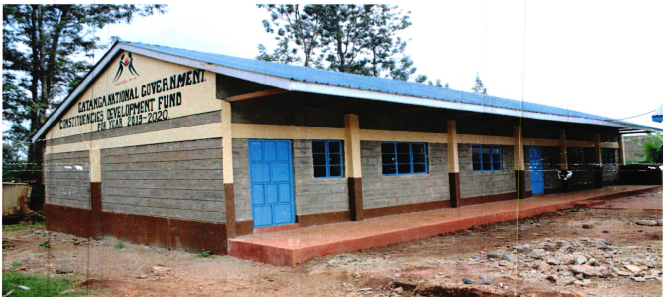
Construction of 2no classrooms at Gatanga Technical & Vocational College
