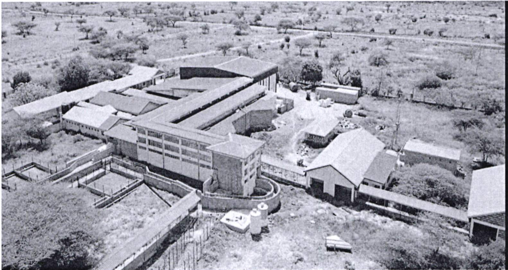
On going Construction of Isiolo Abattoir
