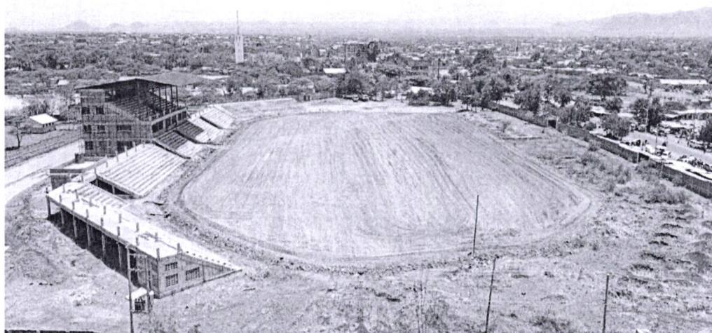
On going Construction of Isiolo Stadium
