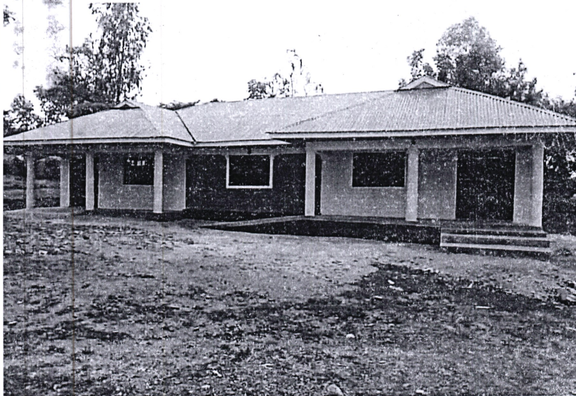
Alara Korayo Primary School Administration block
