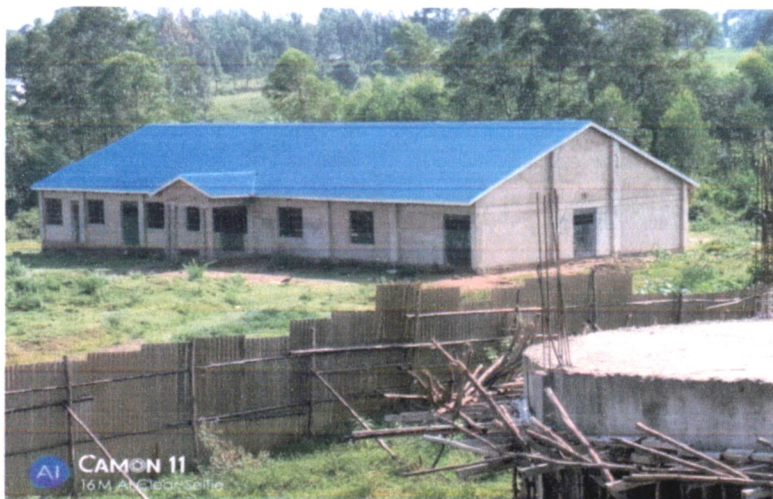
NG-CDF Rongo Sponsored Dining Hall nearing completion.
