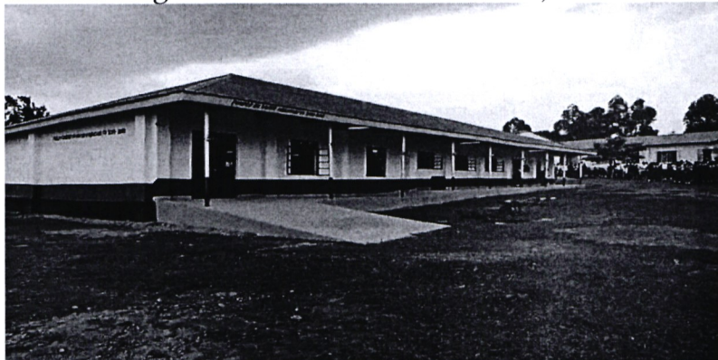
BUSAKALA SECONDARY SCHOOL – CONSTRUCTION OF LIBRARY
