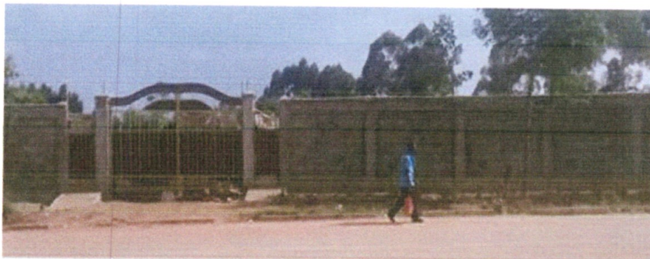
KIMININI PRIMARY SCHOOL UPGRADE OF FIELD GROUND; CHAIN LINK FENCE, PERIMETER WALL 237 METERS, LEVELING AND CARPETING FIELD, RUNNING TRUCK AND ABLUTIONS.
