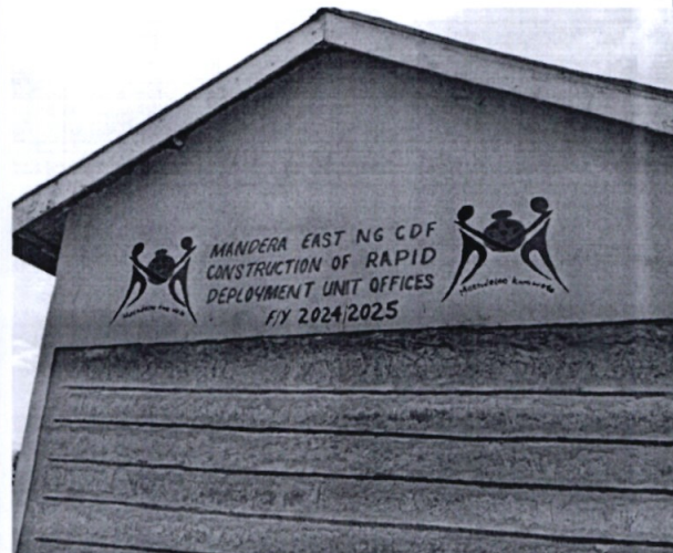
Koromey RDU-Construction of multi-agency offices Impact: Enhanced security in the sub-county
