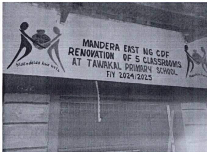
Tawakal Primary school- renovation of 5no. classrooms Impact: improved learning Centres in both primary and Junior secondary school.
