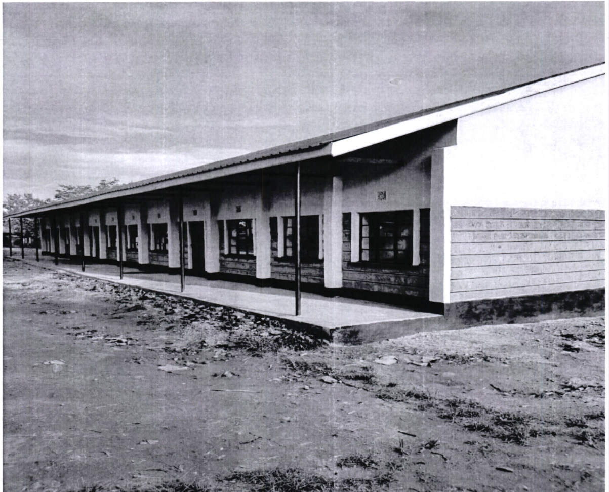
Figure1: Construction of 3 classrooms at AIC Matinyani primary school.
