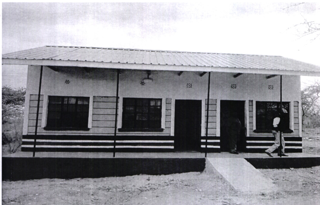
Figure 2: Construction of Chiefs office at Mutanda.
