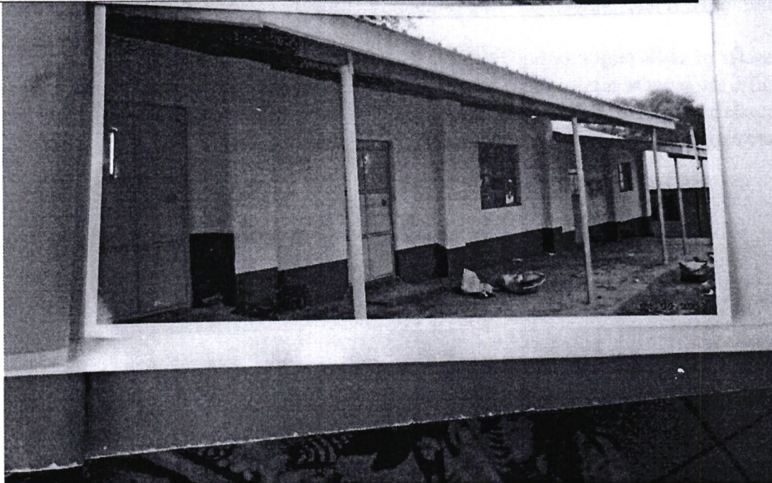
Fig. 5 Mutumbini Primary School classrooms after renovations at Kshs.500,000.00
