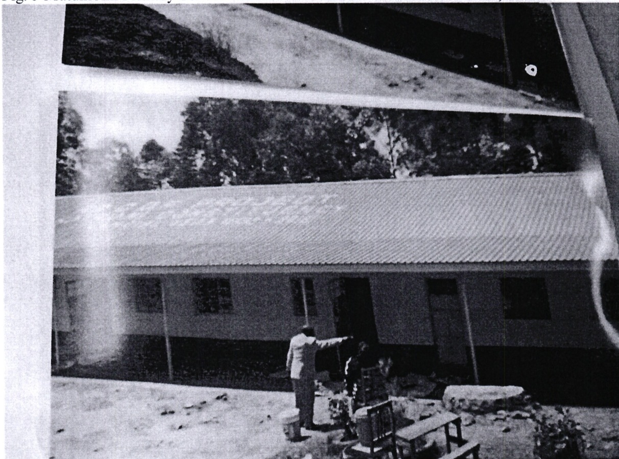
Fig. 6 Kikawani Primary School after renovations at Kshs. 500,000.00
