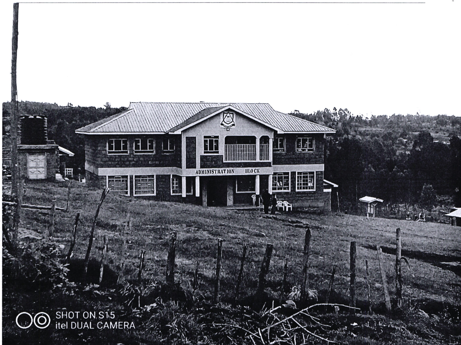
Due to High Need of Education and population, we constructed an administration block at kiheo secondary school to ease congestion of documentation and security of documents as shown in the above diagram in weru ward.
