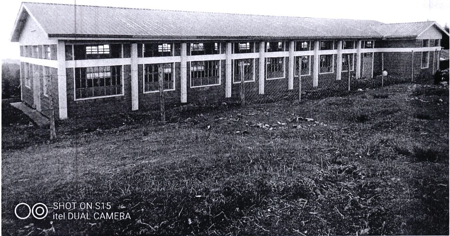
Due to High Need of Education and population, we constructed a multipurpose hall at ruiru secondary school to ease congestion of learner's as shown in the above diagram in charagita ward.
