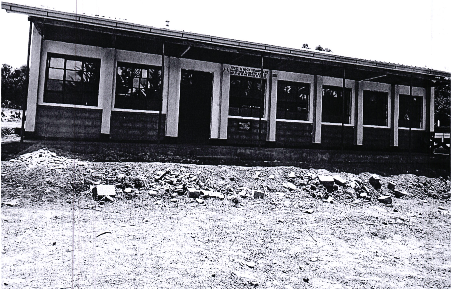
Due to High Need of Education and population, we constructed a laboratory block at gikingi secondary school to enhance smooth education due to increased practical's as shown in the above diagram in gatimu ward.
