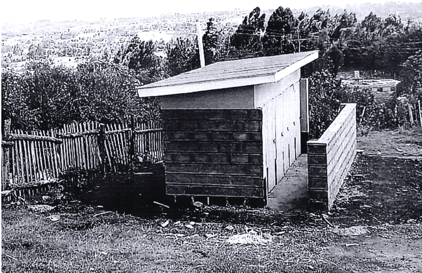
Due to High Need of Education and population, we constructed at 12 door toilets at mahua primary school to ease congestion of learner's as shown in the above diagram in charagita ward.
