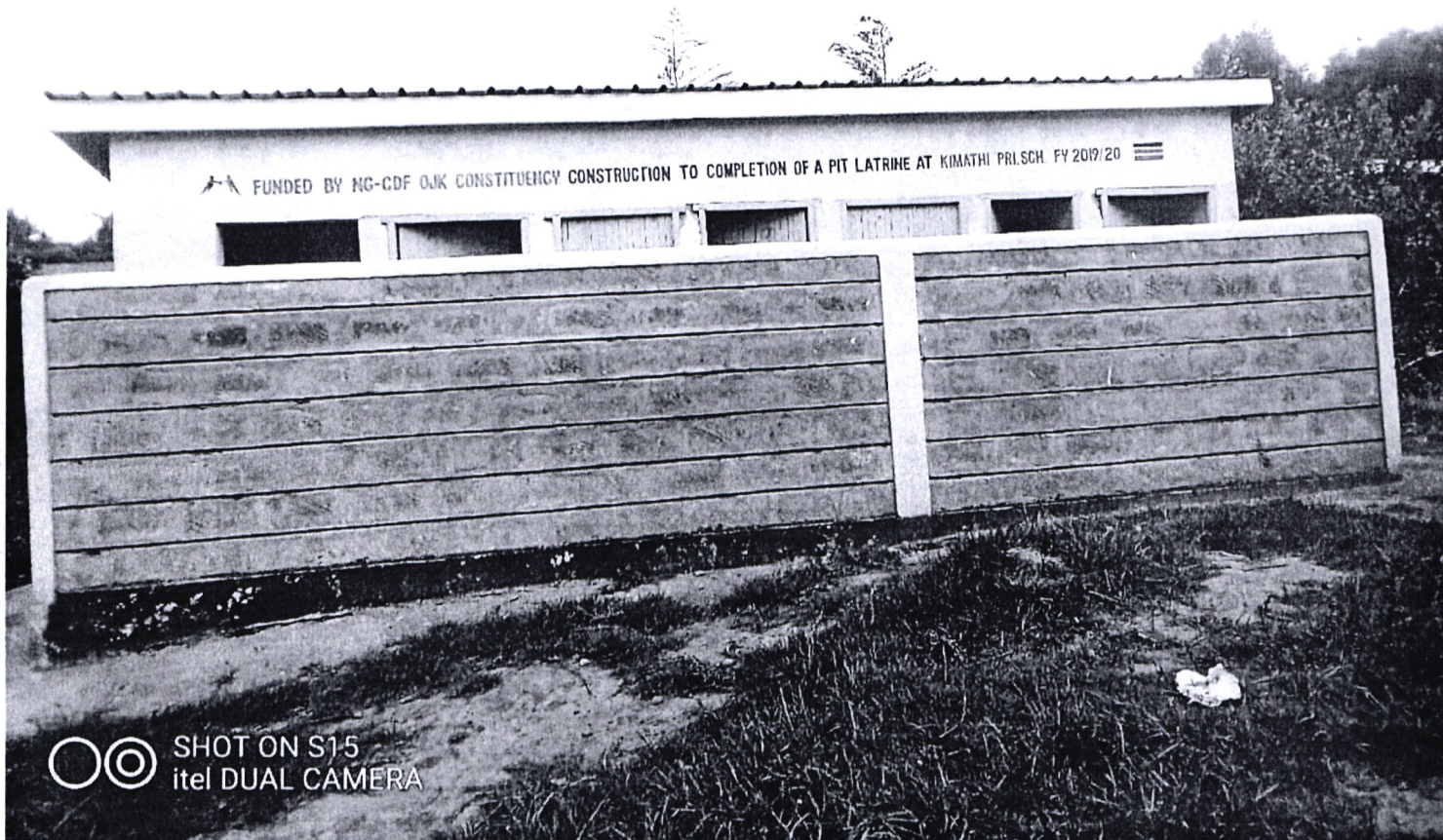
Due to High Need of Education and population, we constructed a six door pit latrine with urinal at kimathi primary school to enhance hygiene as shown in the above diagram in Gatimu ward.
