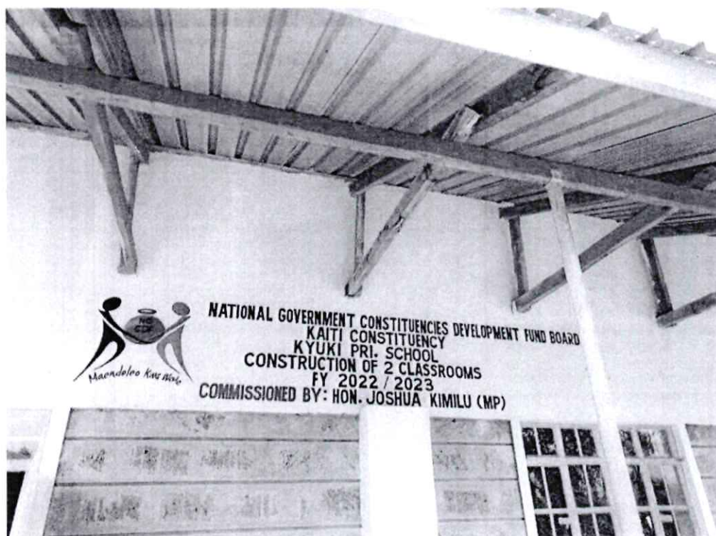
FIG 1: KYUKI PRIMARY SCHOOL-CONSTRUCTION OF 2 CLASSROOMS
