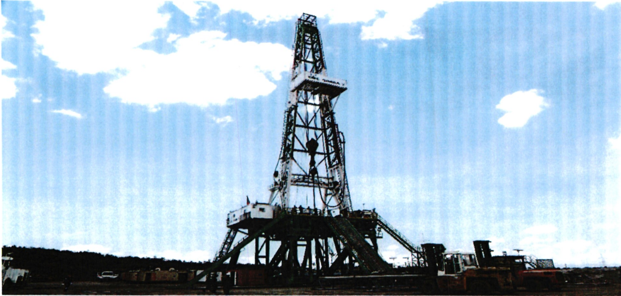
Geothermal drilling rig at Menengai field
