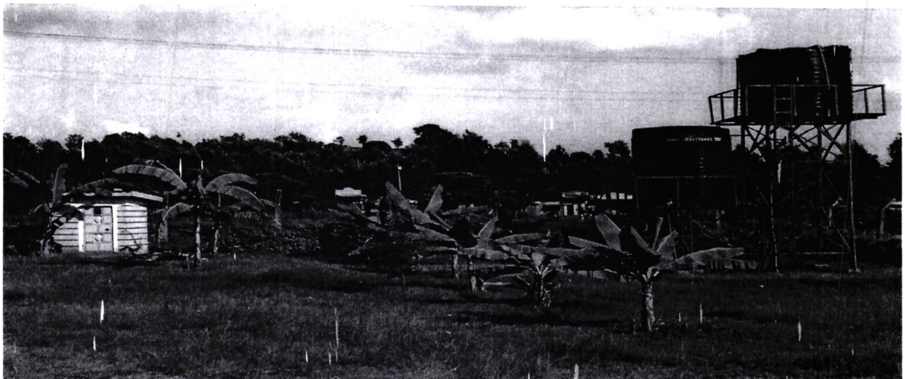
Figure 5-NGCDF office Borehole Project
