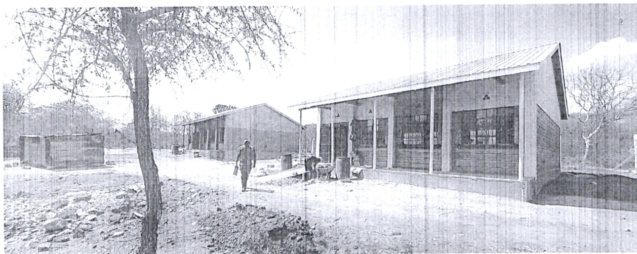
2No. lecture hall construction on-going at Ikanga Teachers Training College
