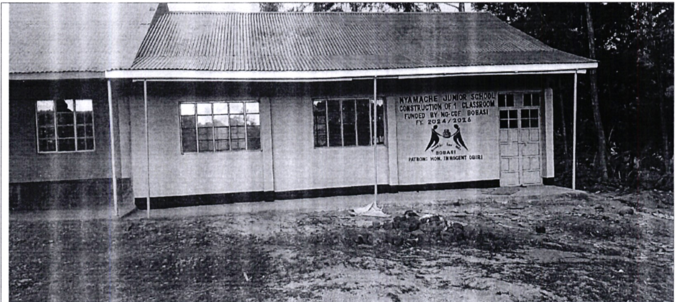
Fig. 2 NYAMACHE PRIMARY SCHOOL – Construction one JSS Classroom to completion
