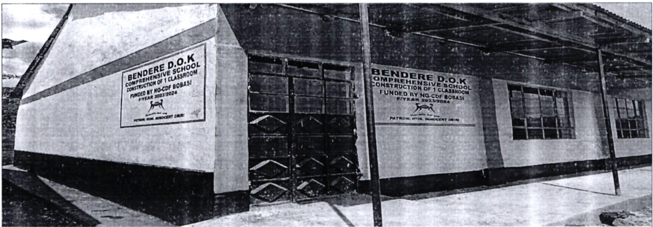
Fig. 1 Bendere Primary School – Construction of one classrooms to completion
