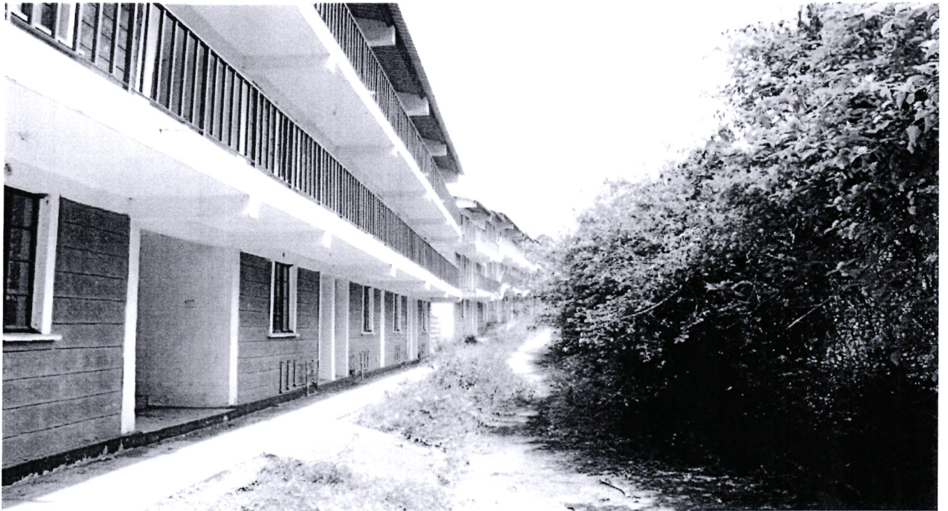
Partially complete House Units in Kibera
