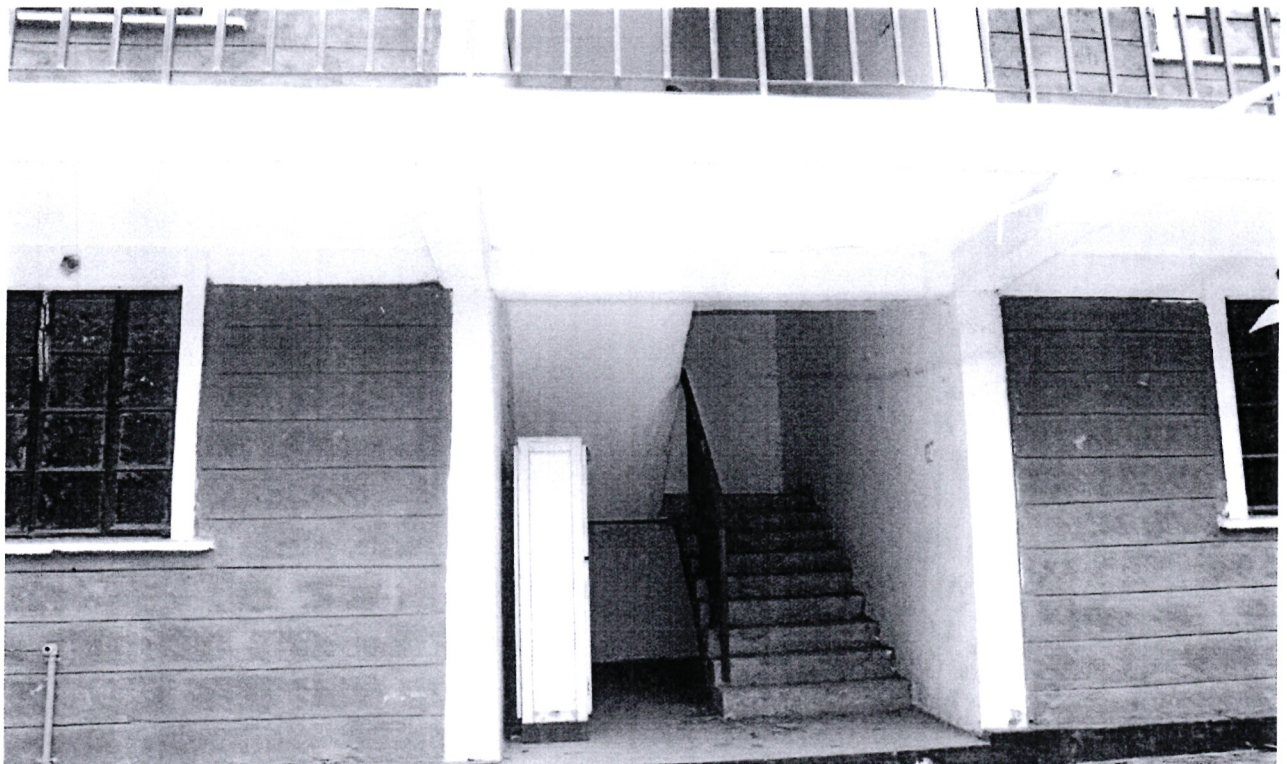
Partially complete House Units in Kibera
