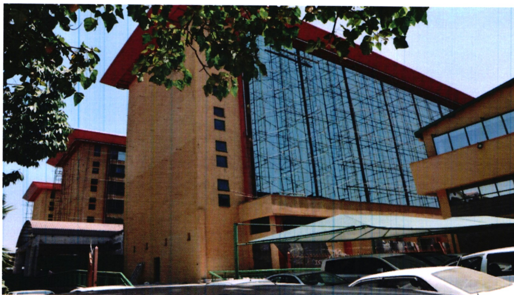
The New Mitihani House (Ongoing Project)
