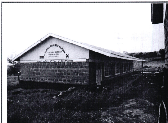
Maraba Primary School-2 Classrooms-Kamara Ward
