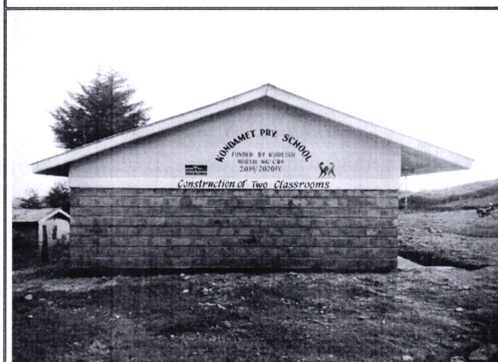
Kondamet Pri School-Construction of two Classrooms-Nyota Ward
