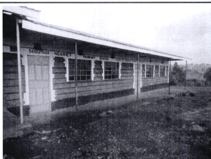
Segutioi Ngariet Pri School-Construction of 2 classrooms-Kiptororo Ward
