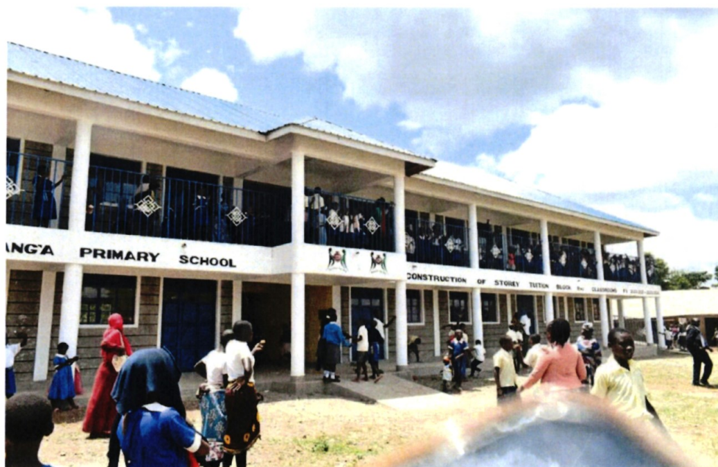
1. Bujwang, Primary School Storey Tution Block
