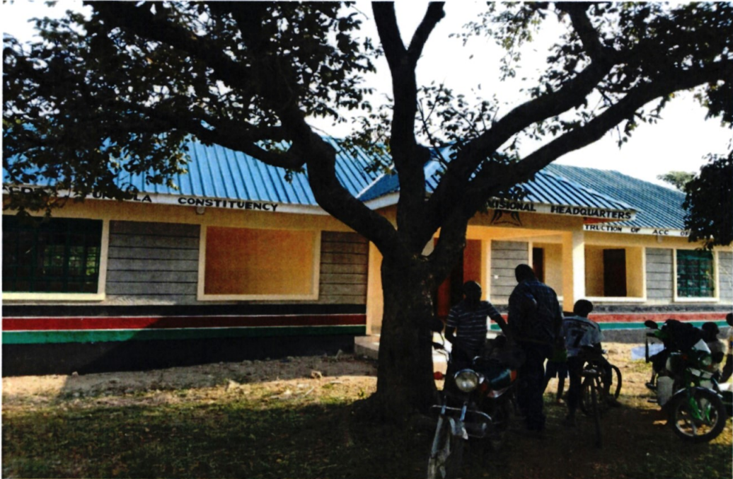
1.Sio Port Divisional Headquarter (Samia Sub County)
