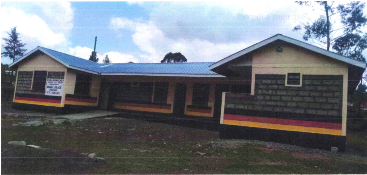
Wanjohi Police Station-Construction of a police station
