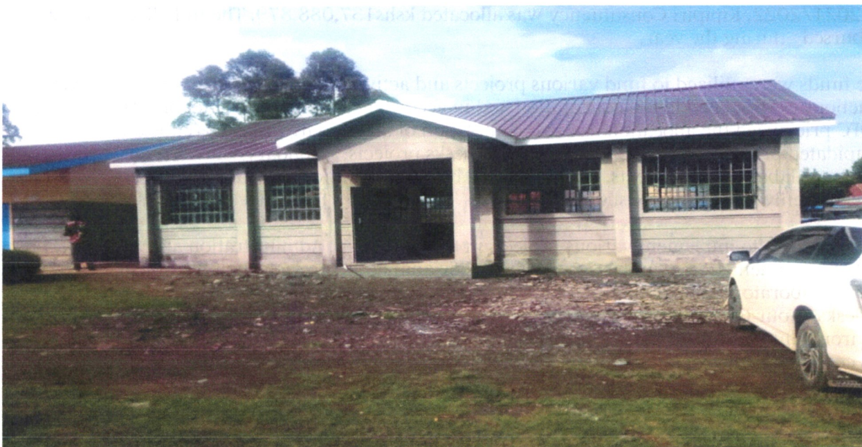
Wanjohi Mixed Secondary School-Ongoing construction of a computer science laboratory
