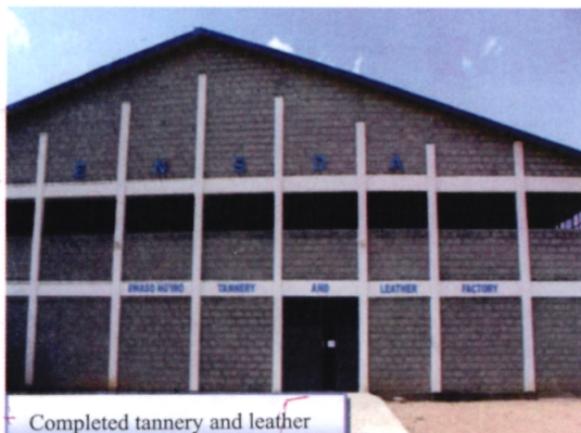
Completed tannery and leather factory building (3,200 m 2 )
