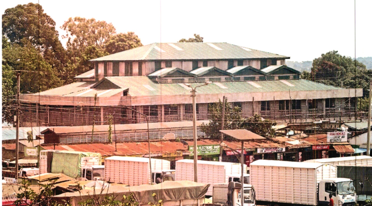
Ongoing Construction of Fish Market (KDSP Project)
