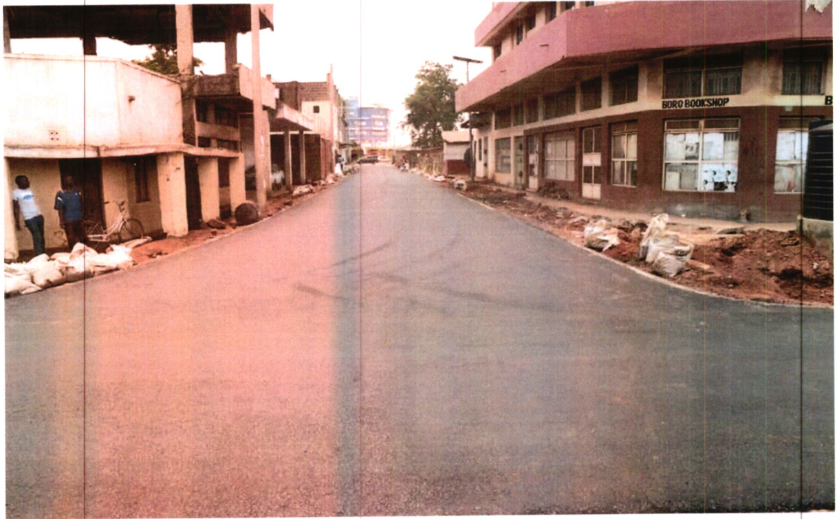
Upgraded Rowcena- Rastopark Road to Bitumen Standard
