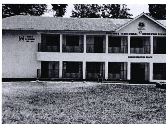
Pic. 3: Construction one storeyed tuition block at Friends Technical Secondary School - Munoywa funded by Sabatia NG-CDF
