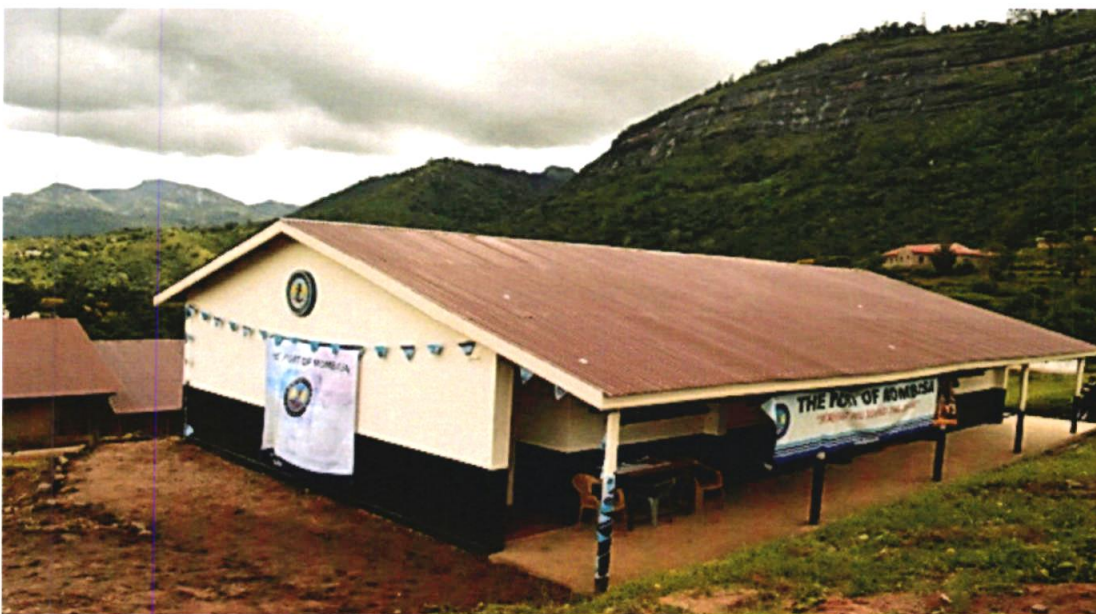
Administration block constructed by KPA at Mwangoji secondary school Taita Taveta County
