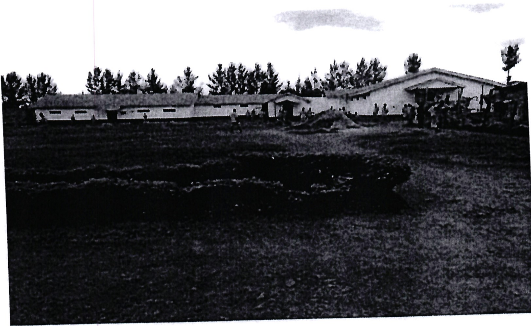
Ngeria prison: Completed Mixed block
