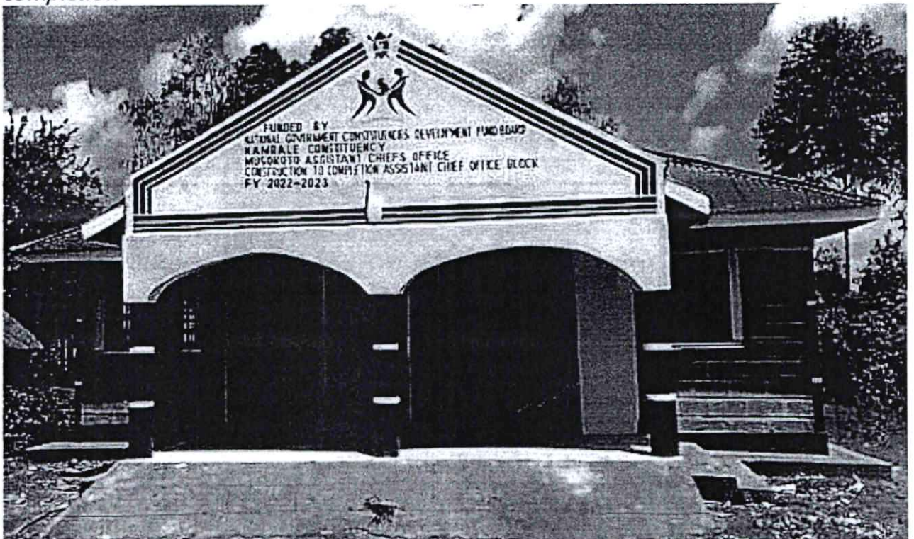
Fig6; Musokoto Assistant Chief's Office-Construction of Assistant Chief's Office to completion
