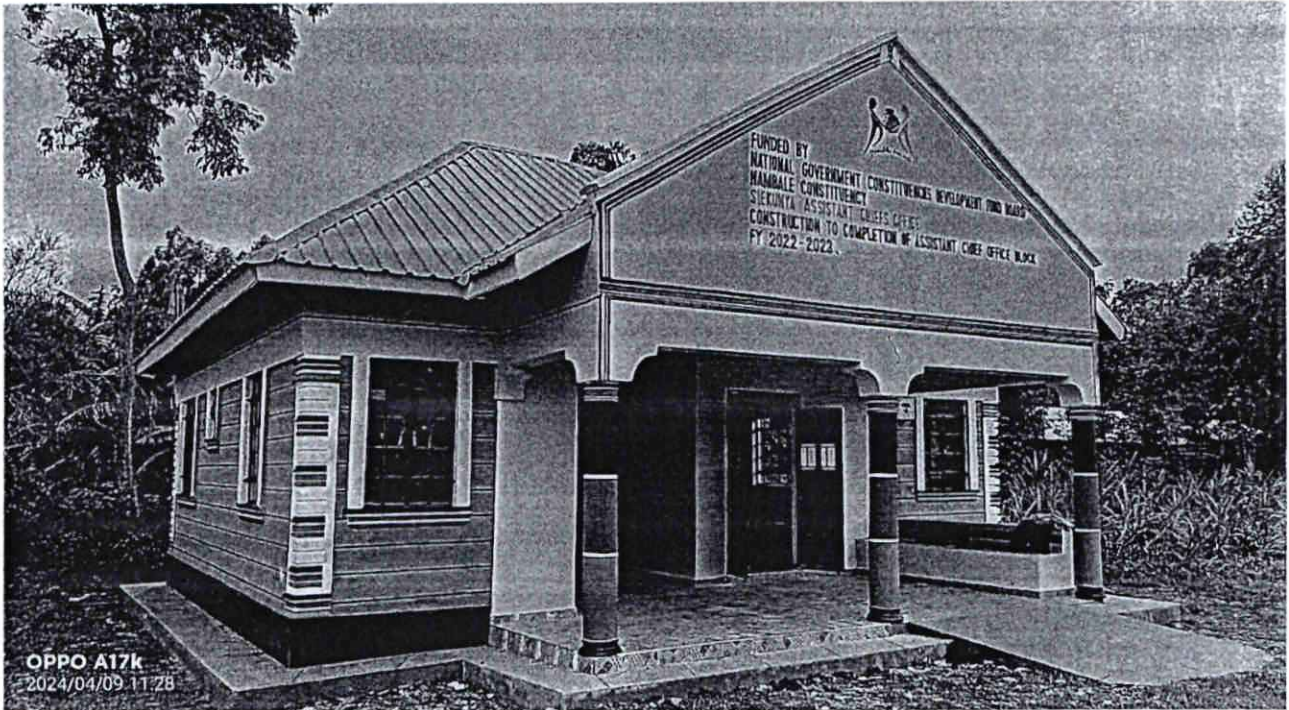
Fig5; Syekunya Assistant Chief's Office- Construction of Assistant Chief's Office to completion
