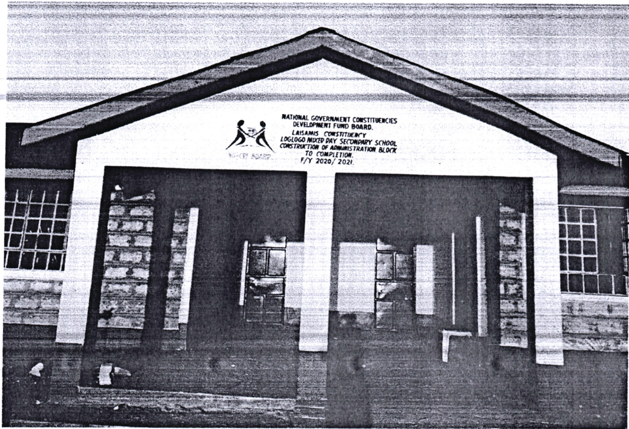
Figure 1: Loglogo Mixed Day Secondary School- construction of administration block to Completion
