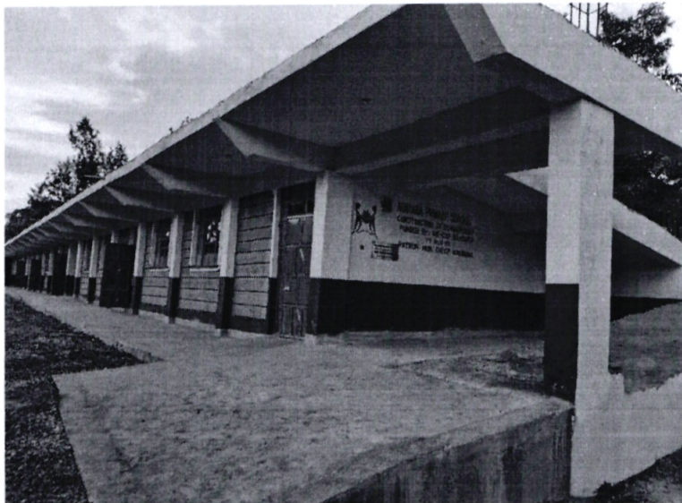
Ngararia primary school construction of 10 classroom block
