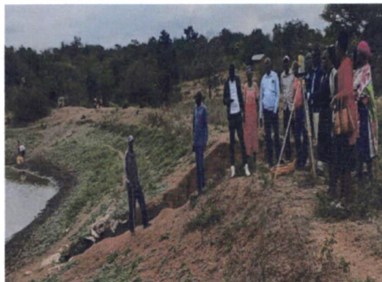
Figure: PMC onsite training ahead of desilting
