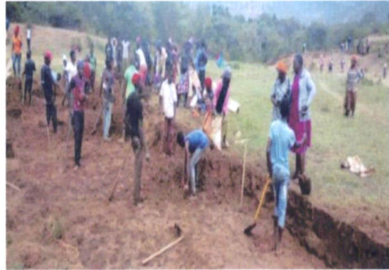
Figure: Desilting of Kyambulu earth dam, Tulumani ward
