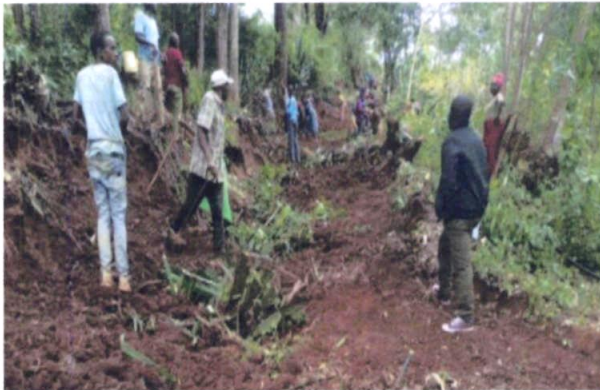
Figure: Gully filling at Kitonguni Cluster Road Project
